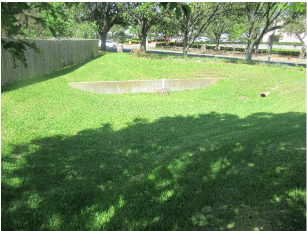
Overview of filtration basin
