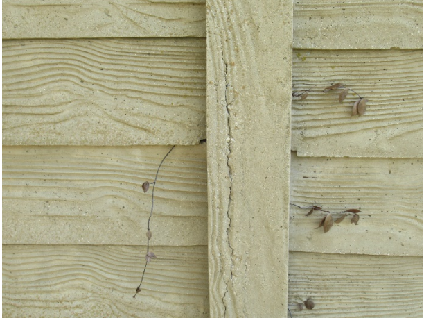
Concrete column crack
