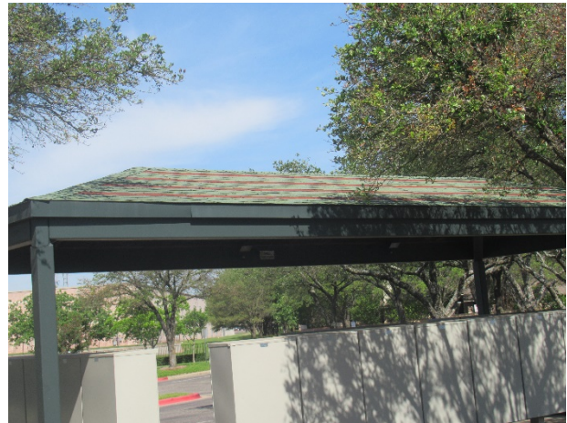
Mailbox kiosk roof
