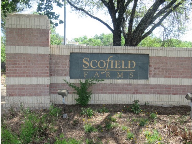
Overview of masonry at monument
