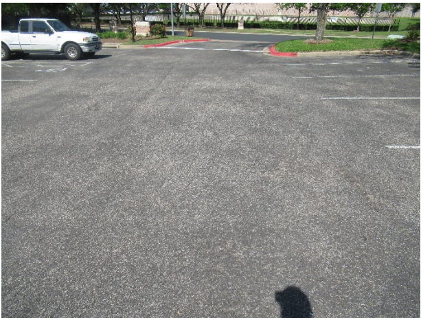
Overview of parking area
