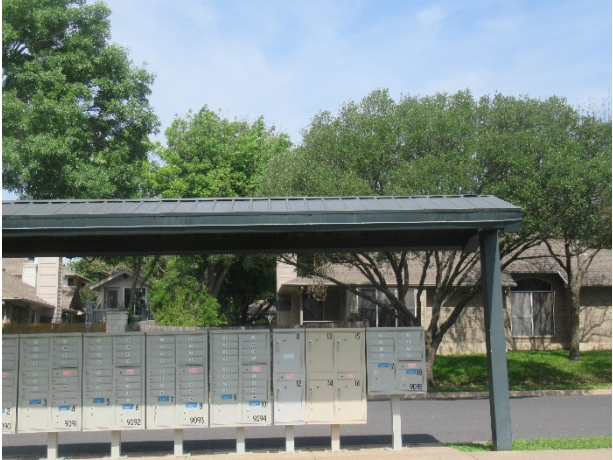
Overview of mailbox kiosk roof
