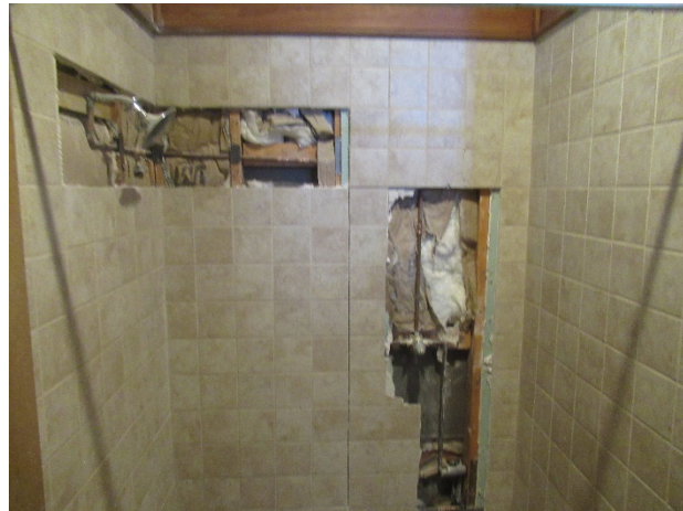
Repairs being performed to pipes
