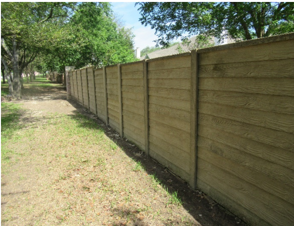
Overview of panelized perimeter wall
