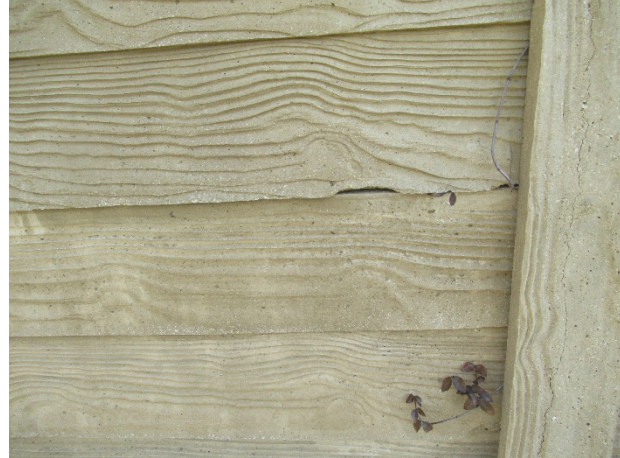
Minor deteriorated concrete
