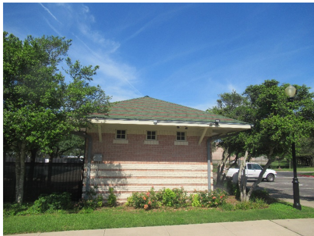
Pool house masonry
