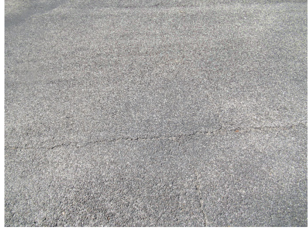
Transverse and longitudinal cracks
