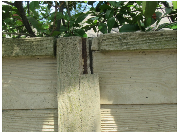
Exposed reinforced steel
